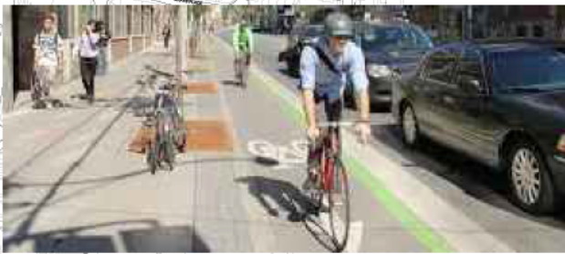
CUT INTO FOOTWAYS TO CREATE SEGREGATED CYCLE TRACK AND NARROW VEHICLE RUNNING LANES
