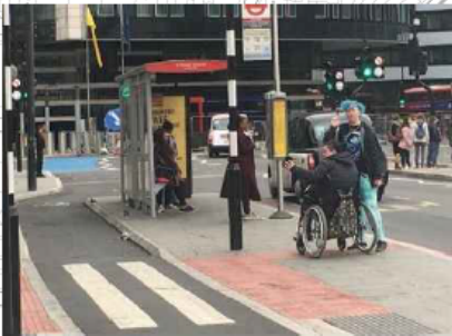
BUS STOP BYPASS CYCLE FACILITY
