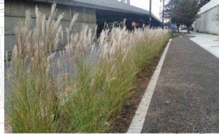
CUT INTO FOOTWAYS TO CREATE SEGREGATED CYCLE TRACK WITH SUDS AND NARROW VEHICLE RUNNING LANES
