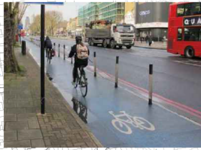
PUBLIC HIGHWAY TO NARROW FOR SEGREGATED PATH. USE OF SEMI SEGREGATION WITH FEATURES SUCH AS ARMADILLOS WITH WANDS
