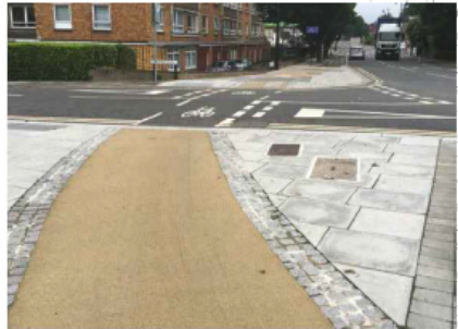
PRIORITY JUNCTION IMPROVEMENTS TO SIDE ROAD.
